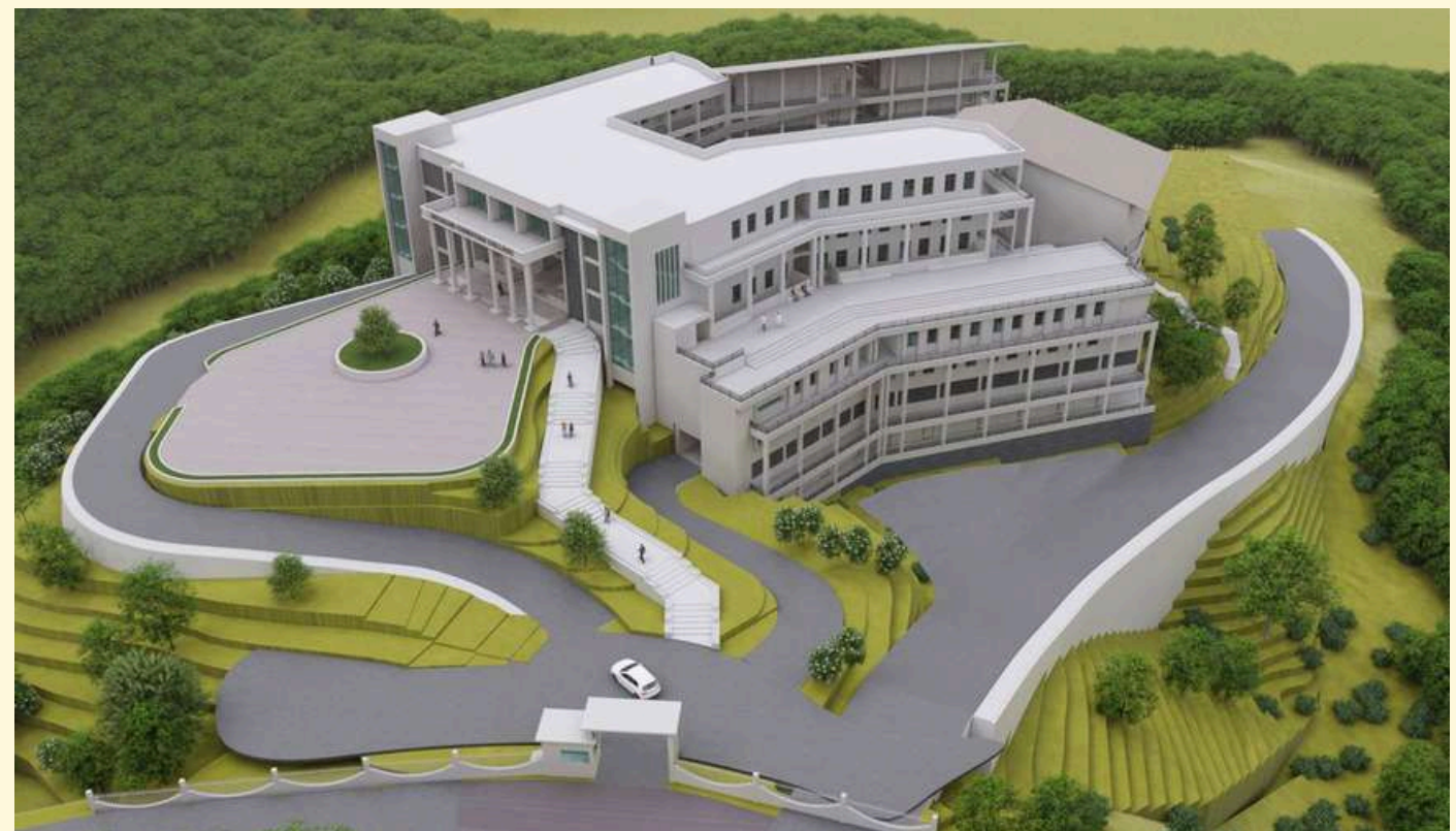
New College Campus under construction at Tanhril
